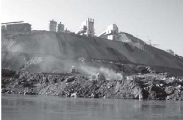
Jinghong Dam under construction
